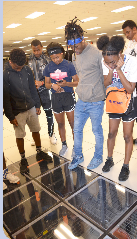
Above: I-STEM campers get a chance to see the access panels beneath the room where the Blue Waters Supercomputer is housed.
